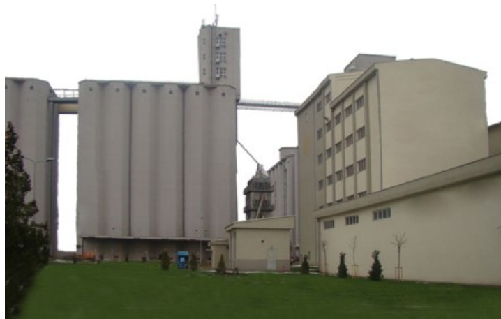
Figure 8. The most suitable facilities for keeping of grainy products for human and animal food are vertical and horizontal silos
